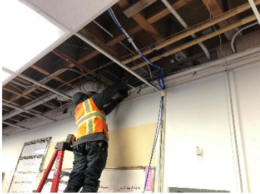
Seismic retrofit & ADA upgrades
