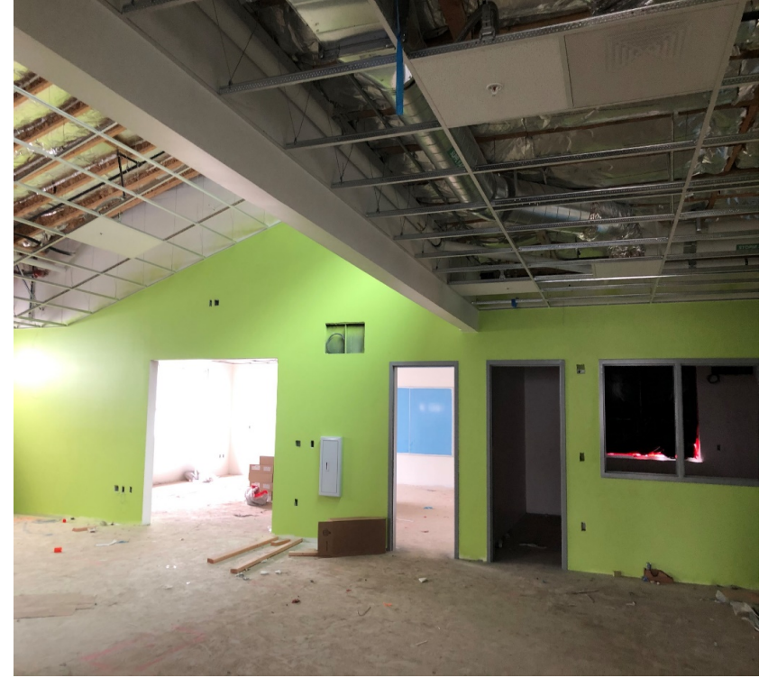
Learning Suite South with Paint Ceiling
