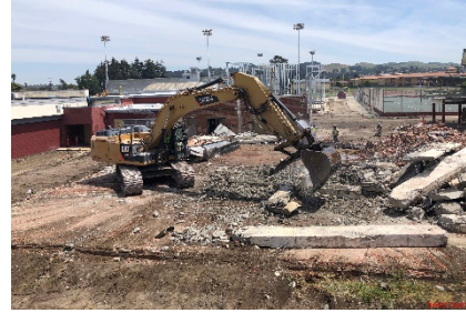
Demolition of the old dance room & locker room which will soon be a new quad
