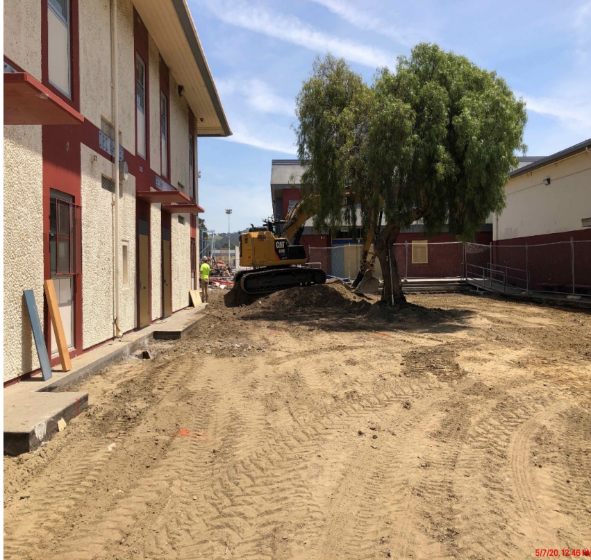
Science Quad Paving Removed
